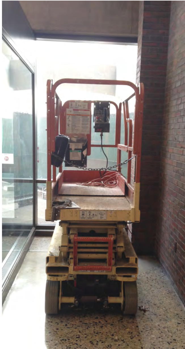
Fig 77 | above. The scissor lift used for installation
